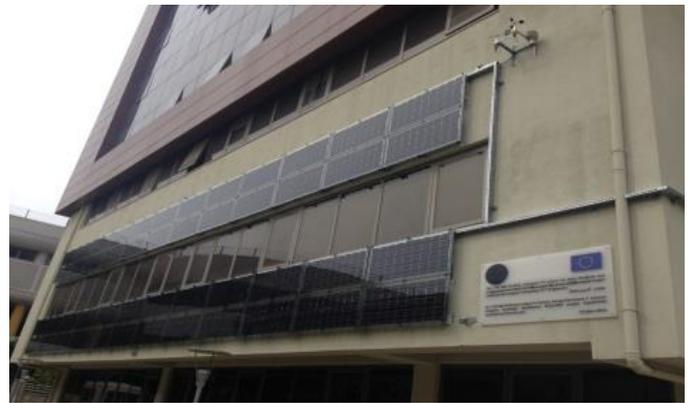
Figure 2. Experimental BIPV system installed on the southeast façade of building Y
